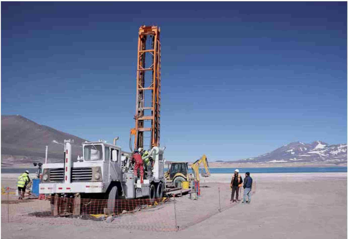
Site of the perforations in the Laguna Verde project.
