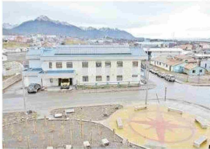
Hospital Cristina Calderón de Puerto Williams.
