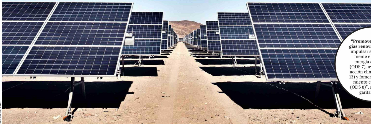
ENEL GREEN POWER
